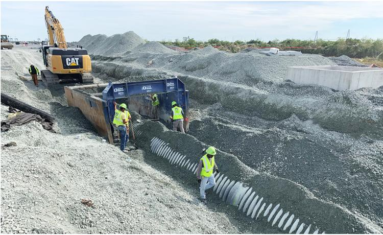
of the redesign, some 27,000 feet of ADS HP Storm pipe in diameters ranging from 12 to 60 inches in diameter was used to convey all storm water on the 280-plus acre site. Distributor, Ferguson Waterworks, handled the logistics of providing the pipe, fittings, and other required components on a just-in-time basis.
